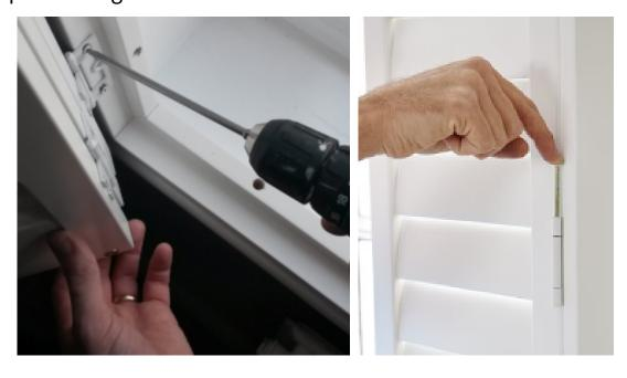
When you are happy with your panel alignment, insert the small hinge screw into the round hole on the hinge to lock them in position.
